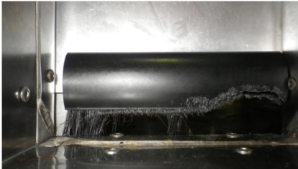
Photo 20 Condition of control sample installation after 2 days (Cycle III) - Entry into feed station
